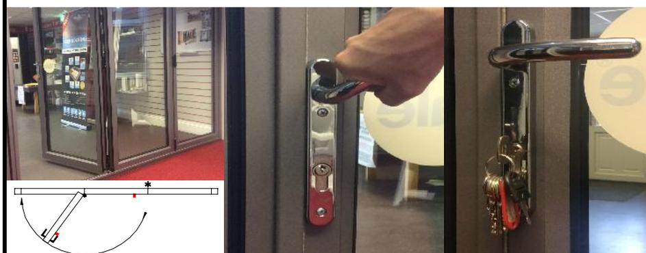
Release the traffic door from the magnets (if fitted) and close
